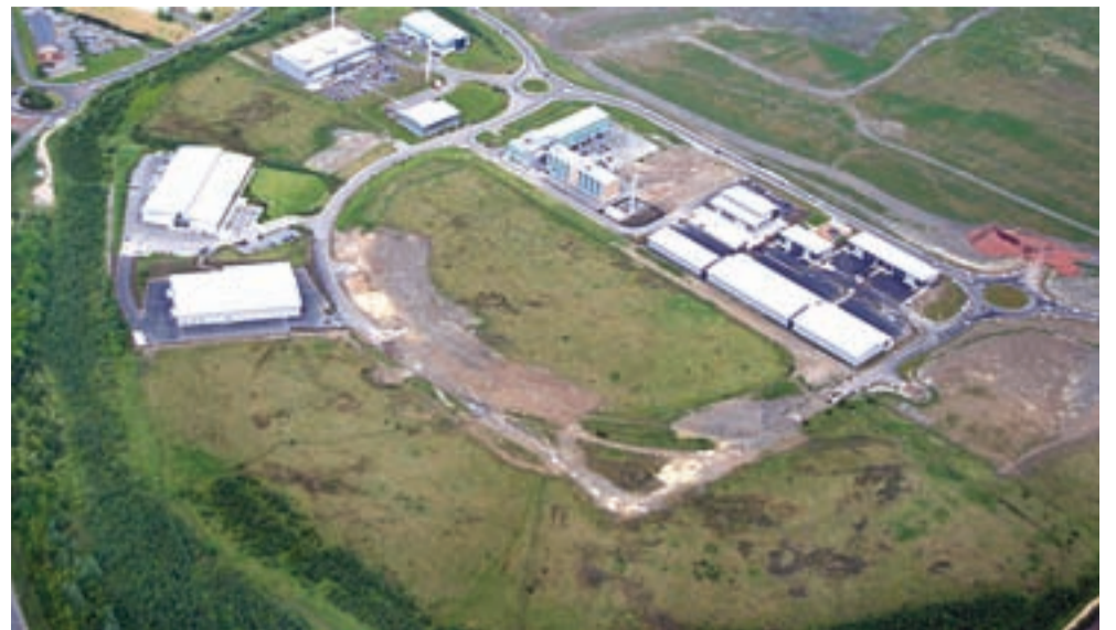
FLYING THE FLAG: The Advanced Manufacturing Park is one of the world's leading hubs for research and development, innovation, manufacturing and engineering
