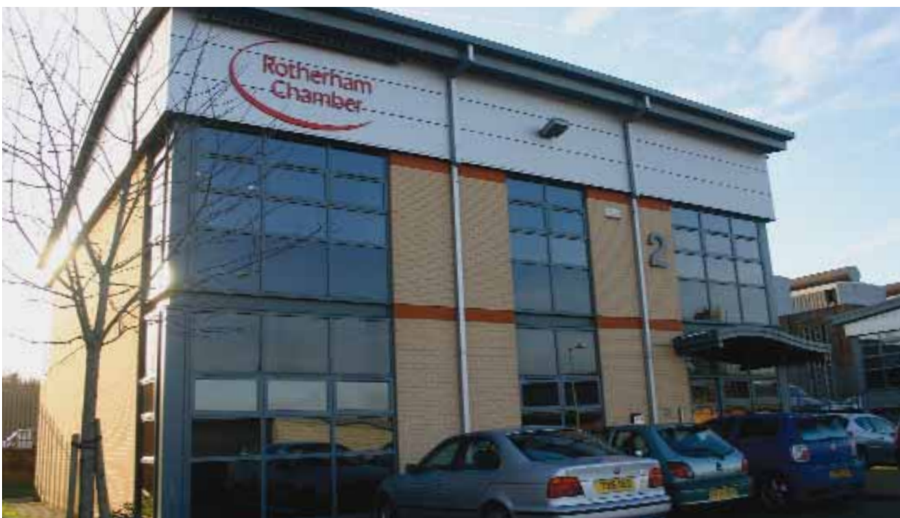
The new Rotherham Chamber HQ at Templeborough, Rotherham
