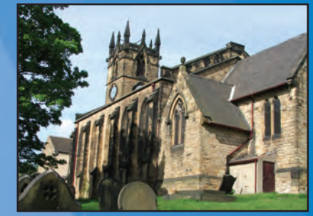
Figure A: ST Thomas' Church seen from the footpath
