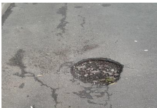
Carriageway Pothole deemed Cat 1 by the Highway inspector using the Risk Based Approach
