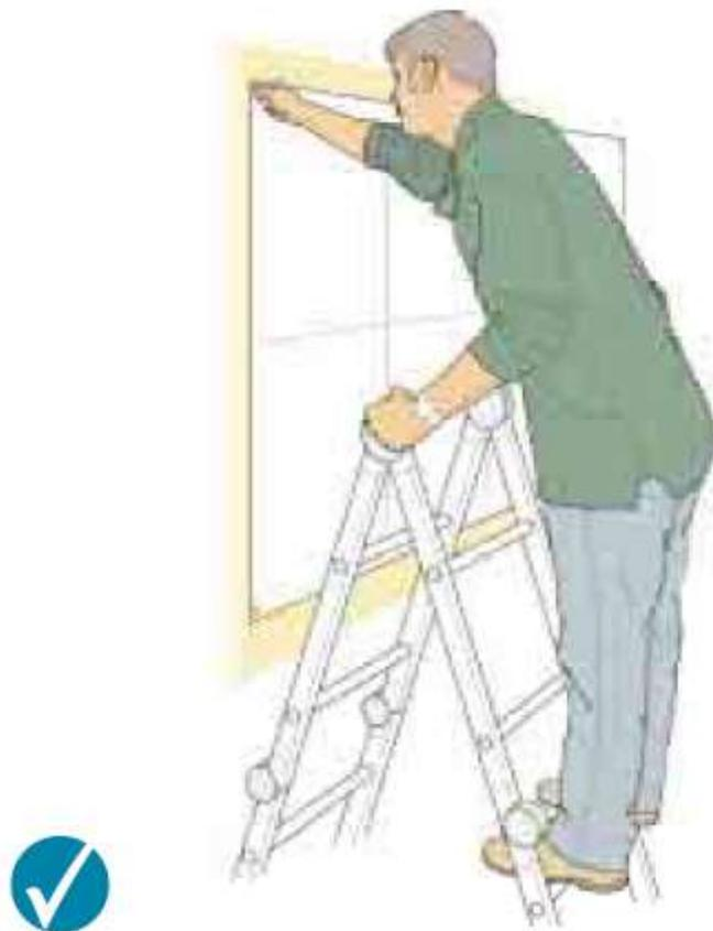
Figure 11 *Correct - two clear rungs. Don't work any higher up this type of stepladder*
