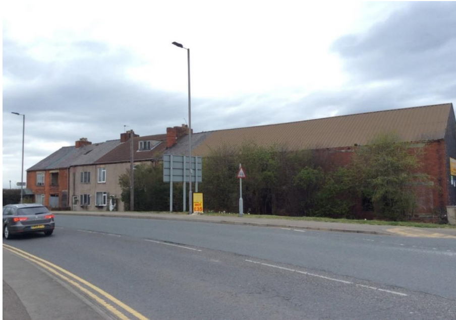
Derelict building formerly in business use
