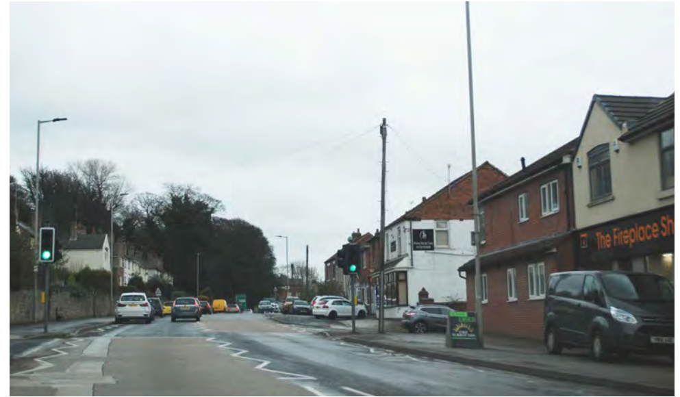
Parking dominated frontages on the west of Maltby
