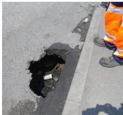
Lighting Column access cover Carriageway Collapse Missing Chamber Cover Removed exposing cables
