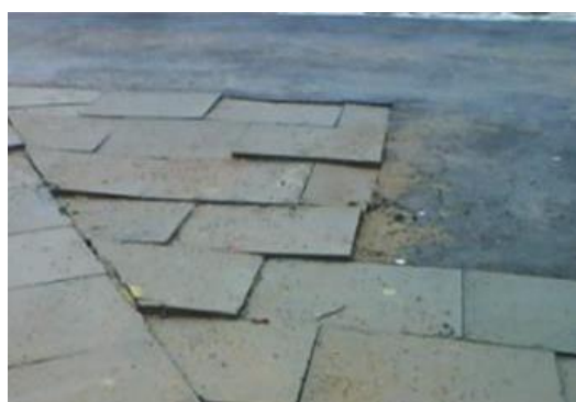
Uneven flagged Footway and potential tripping hazard
