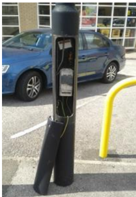
Lighting Column access cover Carriageway Collapse Missing Chamber Cover Removed exposing cables
