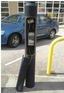
Lighting Column access cover Removed exposing cables
