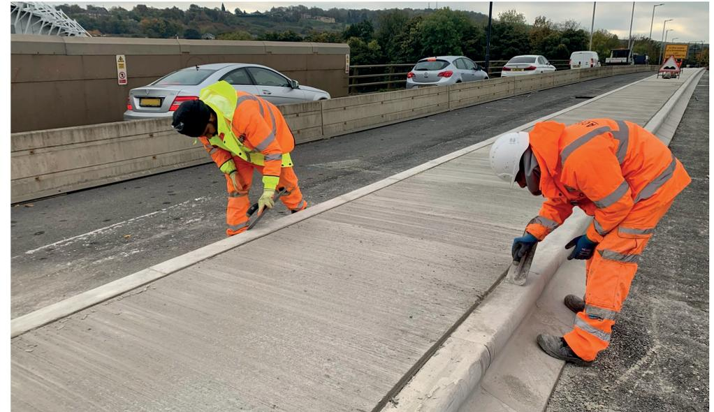
The project team prioritised a solution that minimised disruption to the highway while addressing safety concerns. This involved securing the expansion joints in two sections and fixing 140 slabs with enhanced security. A safety system was installed to protect the central reservation, and the carriageway was resurfaced.
