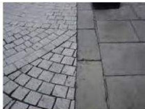
Fan shaped concrete cobbled carriageway with original yorkstone pavements on Church Street.
