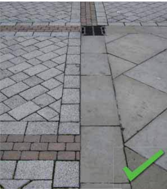
The paving in the Town Hall Square as seen above is tidy and well thought out, from the placement of the drain to the transition of materials.
