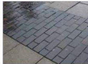
Clay pavers are a slip hazard in some locations.
