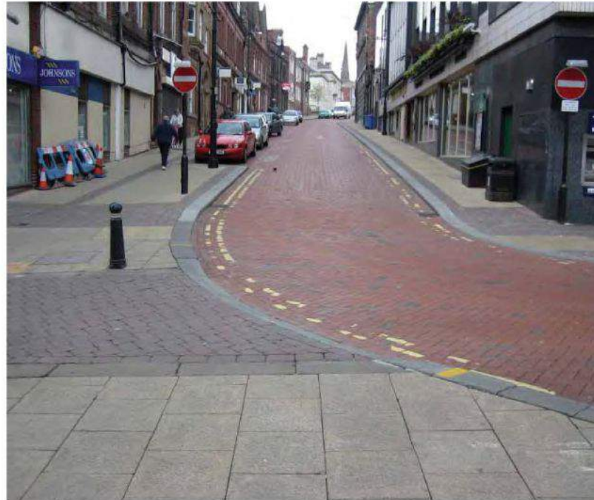
Use of seven different surface materials at junction are conflicting creating a disharmonious public realm. Yellow lines appear to be failing on the red pavers.
