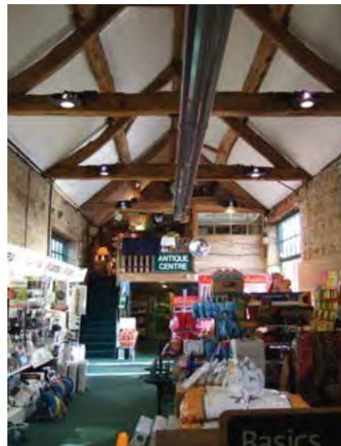
Figure 8 Roof structure of the Grade II listed cartshed
