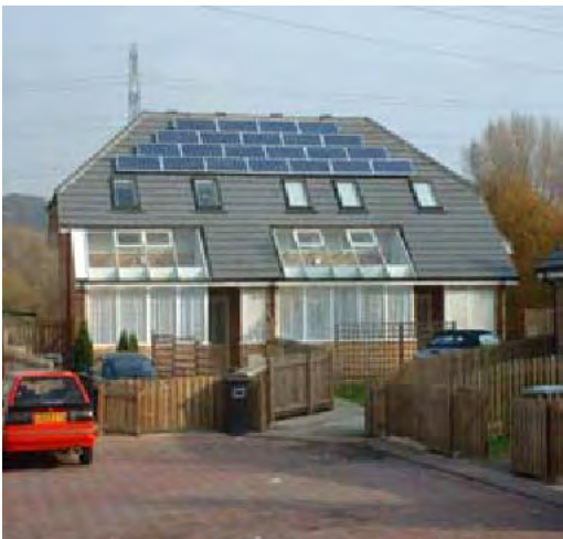
Figure 39 A PV installation at Sackville Street, Ravensthorpe, in Kirklees. (Source: Renewable Energy Initiatives In Kirklees, Kirklees Metropolitan Council, September 2005)
