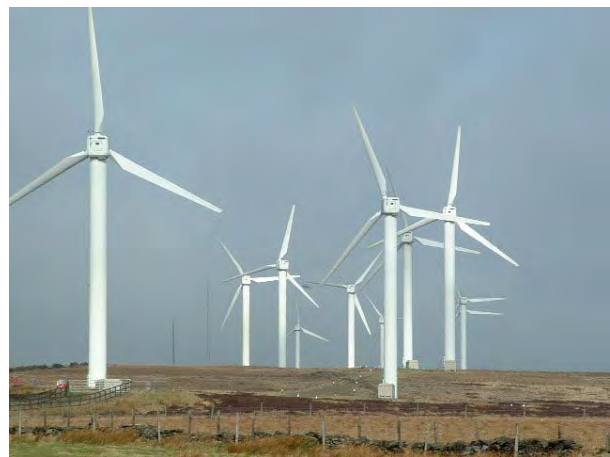
Figure 19 The 9 MW, 23 turbine, Ovenden Moor Wind Farm in Calderdale. This wind farm has been operational since 1993 and an application has been submitted to planning for repowering of the site with larger turbines. (Source: Nigel Homer, March 2005, retrieved from Wikimedia website, accessed November 2010)
